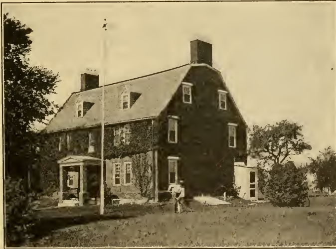
THE CRADOCK HOUSE (1636) AT MEDFORD. This is the oldest brick house in the United States. With the exception of the porch it is in the same condition as in colonial times. Cradock was the first governor (president) of the Massachusetts Company in England. He never came to America, but he did try for a time to till some large grants of land there by bands of indentured servants. These grants were made him in recognition of his services in England.
